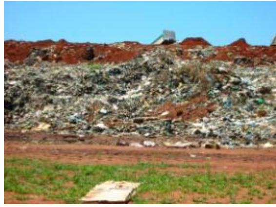
Figure 16: Side slopes not shaped and covered
