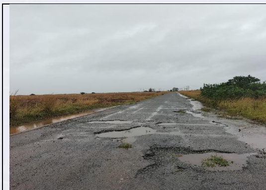
Figure 58: East Avenue state
