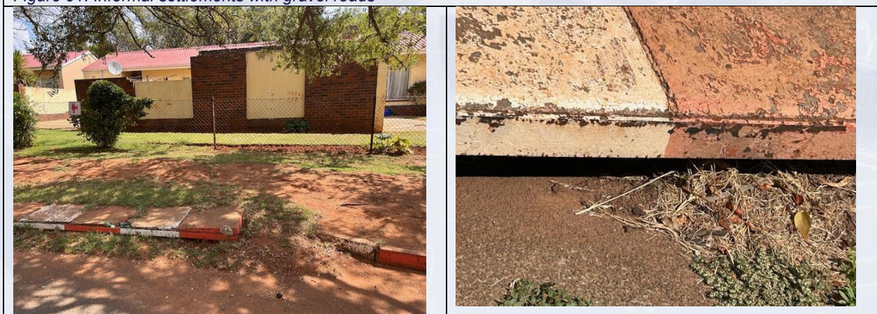
Figure 92: Kerb inlet need cleaning and replacement of covers
