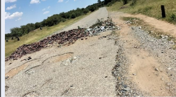
Figure 8: Washed away culvert on Alfred Kobi street
