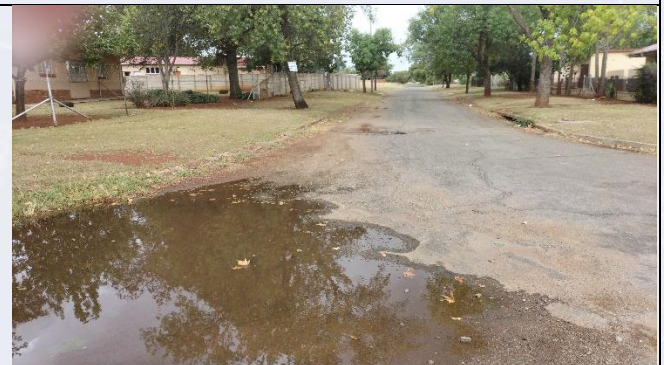
Figure 55: Poor Stormwater management
