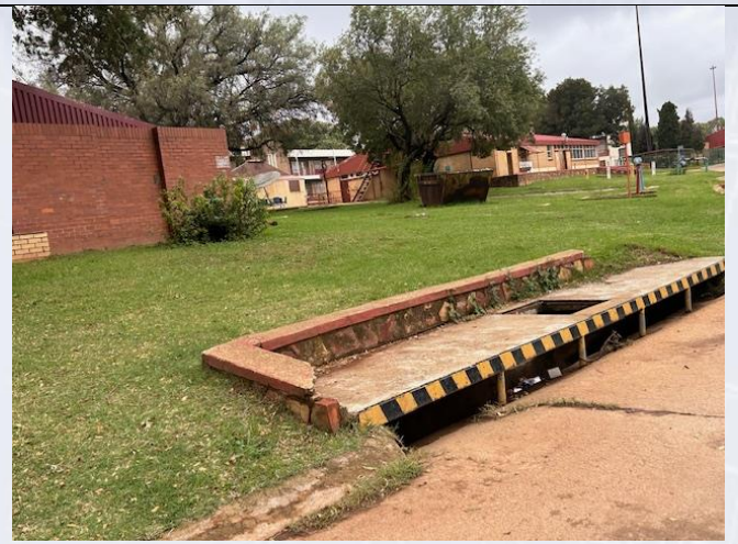
Figure 101: Stormwater kerb inlet
