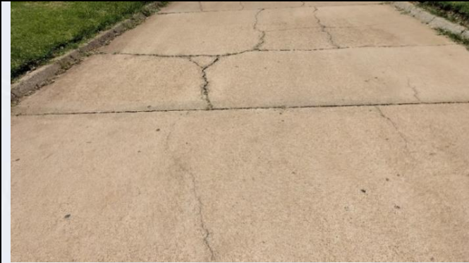
Figure 71: Condition of concrete pavements Photograph 1
