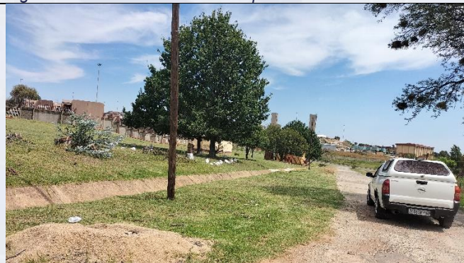
Figure 73: Open channel drain
