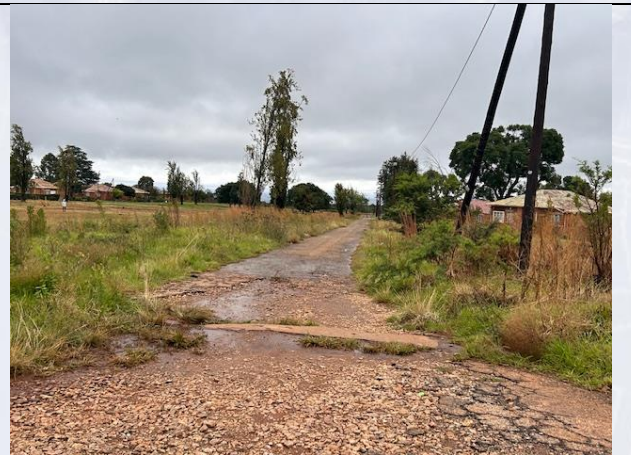
Figure 107: Very narrow street
