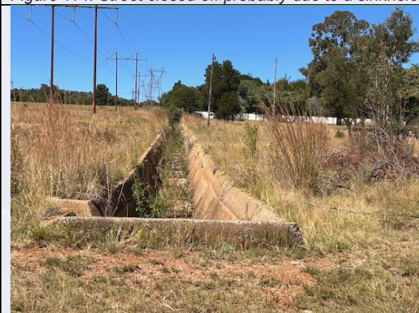
Figure 116: Stormwater channel and junction box
