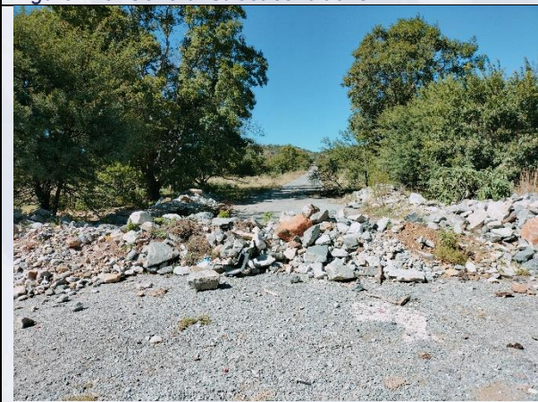
Figure 114: Street closed off probably due to a sinkhole
