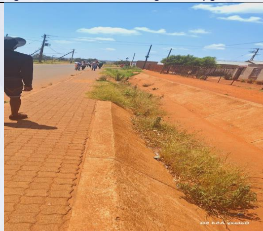
Figure 20: Stormwater drainage-lined trapezoidal open channel
