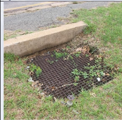
Figure 100: Grated inlet at the entrance into WDLs
