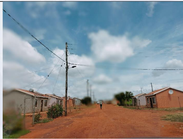
Figure 69: Gravel roads where there are new RDP roads
