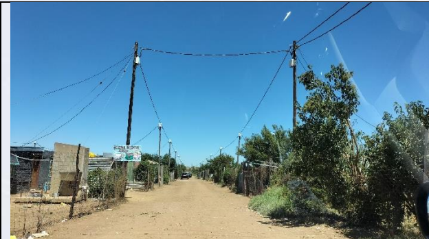
Figure 25: Informal settlements gravel roads
