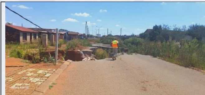
Figure 16: Sinkhole in Khutsong North
