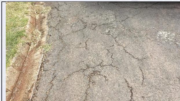
Figure 47: cracked surface
