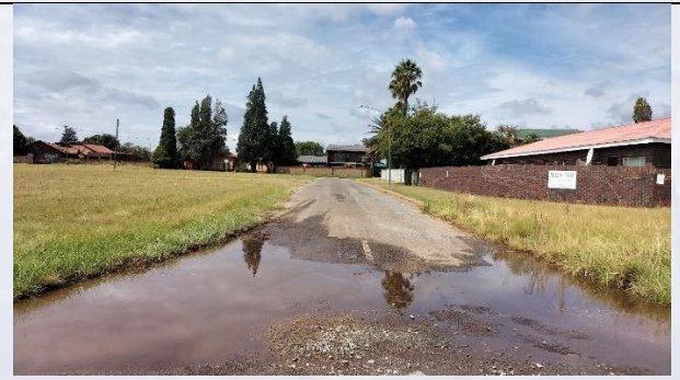
Figure 68: Poor stormwater management Welverdiend South
