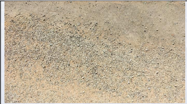
Figure 35: Evidence of surface corrugation
