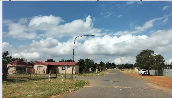
Figure 83: Minor road into Letsatsing
