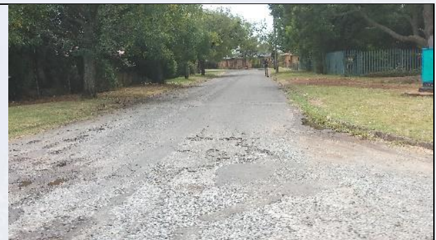
Figure 48: corrugated surfaces
