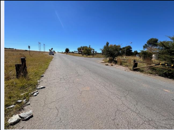
Figure 113: General Street conditions
