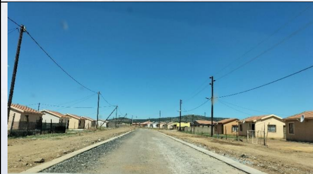
Figure 27: RDP Houses roads being constructed
