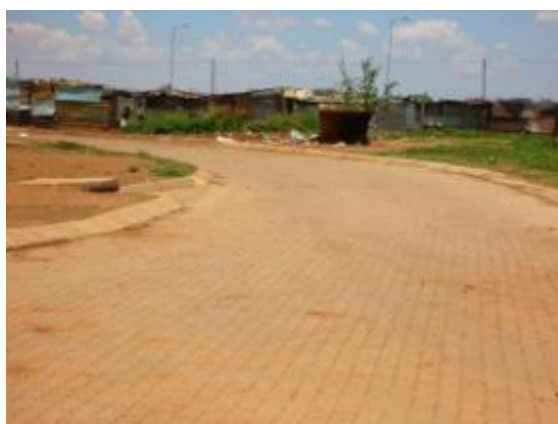
Figure 25: Paved roads in Green's Park
