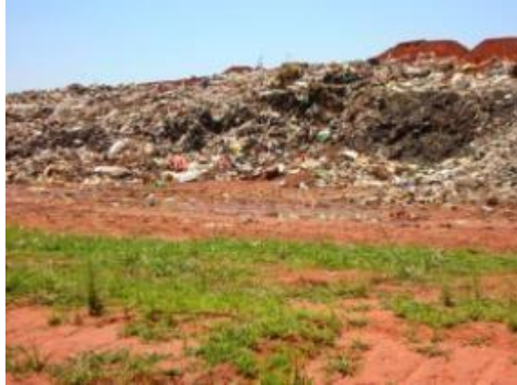
Figure 15: Water ponding at the Rooipoort Landfill Site
