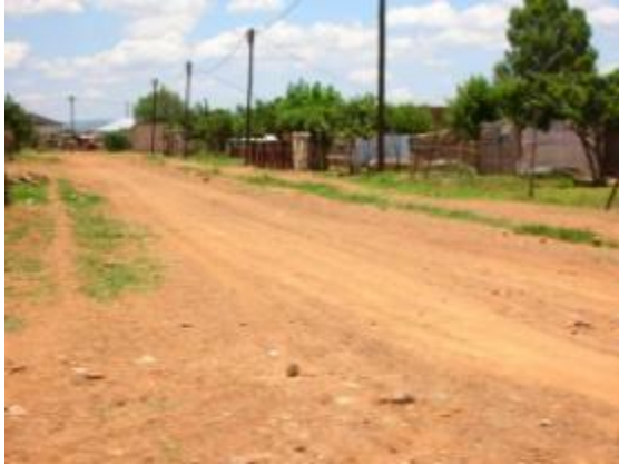
Figure 19: Roads fairly accessible
