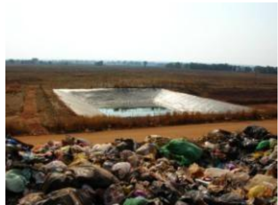
Figure 18: Contaminated water pond
