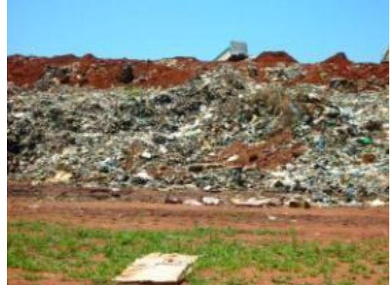
Figure 16: Side slopes not shaped and covered
